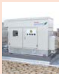
LPG-powered emergency generator
