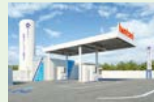
Hydrogen-refueling stations for FC forklifts
